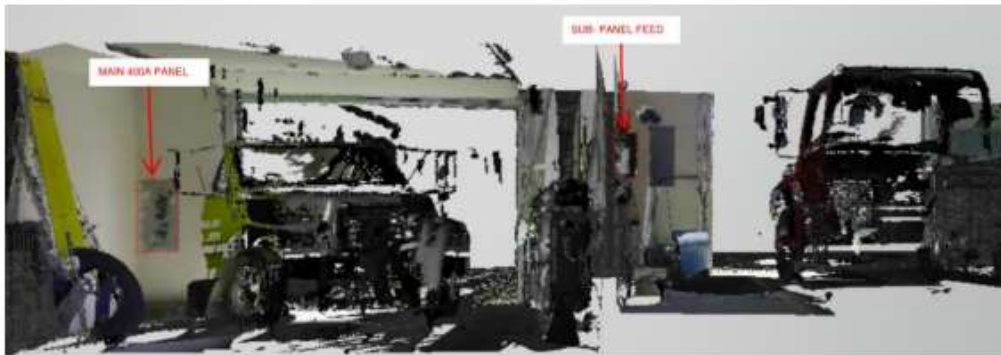
Figure 17 Panel Locations - 132 1st Street, Tulameen
