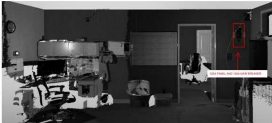
Figure 14 Interior Panel Location - 1109 Willow St
