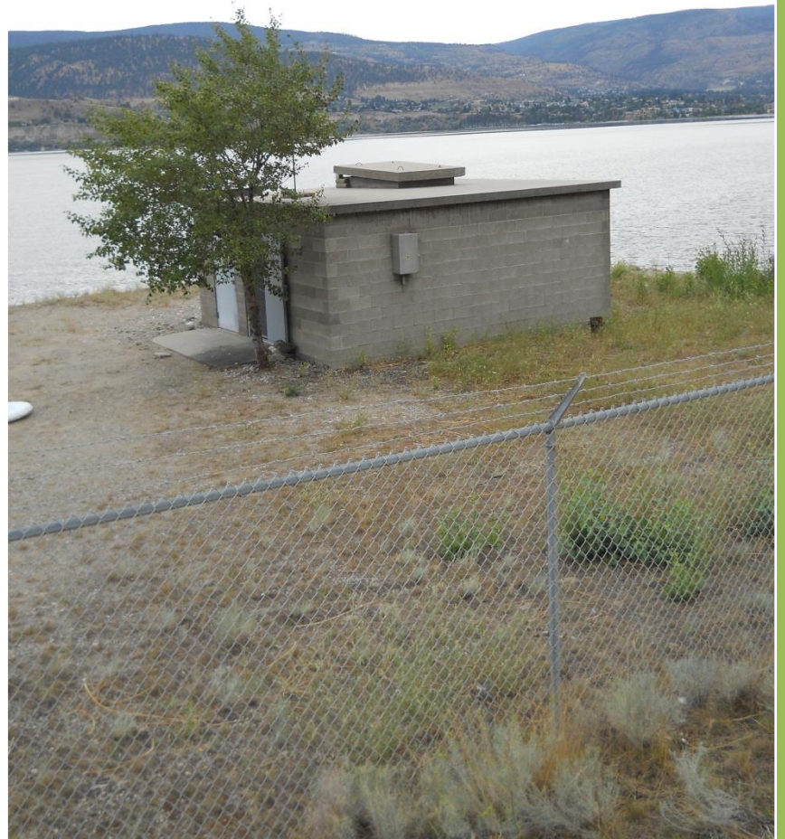
Sage Mesa Lake Pump Station
