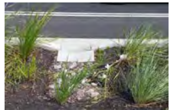
Image 2: Inflow detail showing rip rap splash pad to help prevent erosion
