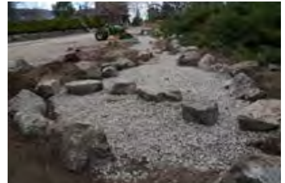
Image 4: Dry creek bed was filled with gravel and large rocks were selectively positioned
