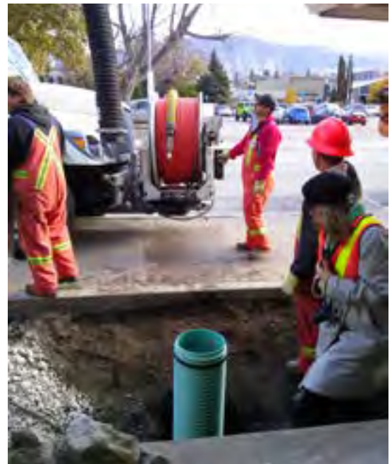
Image 3: Installing the well casing
