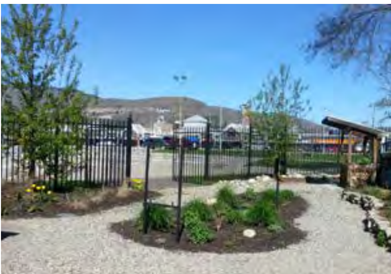
Image 5: Rain gardens after installation
