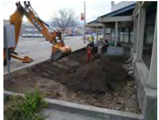
Image 2: Removal of all plant material
