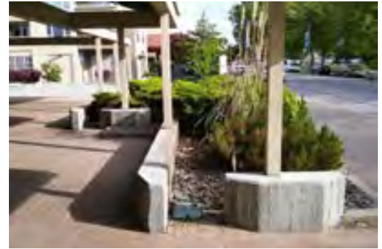
Image 1: Entrance garden overtaken by juniper
