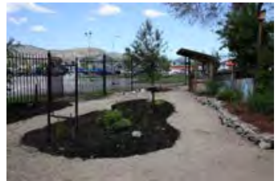
Image 2: After site rehabilitation and rain garden installation
