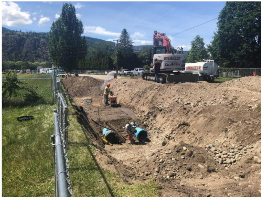
Watermain burial and compaction.
