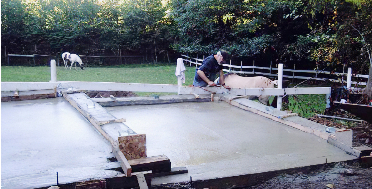
Figure 17. Constructing the concrete slab base using forms 39
