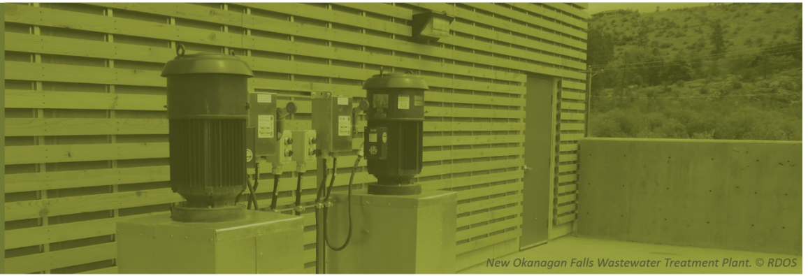
New Okanagan Falls Wastewater Treatment Plant. © RDOS
