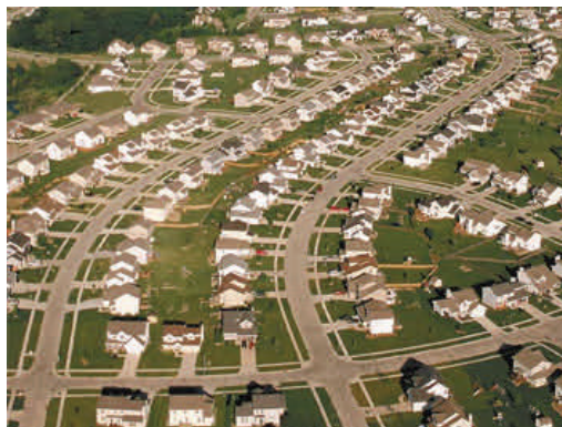
If unchecked, development can have serious consequences on the environment, infrastructure, and, ultimately, on quality of life.
