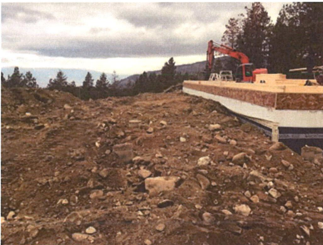
Rough Grading around buildings and site.
