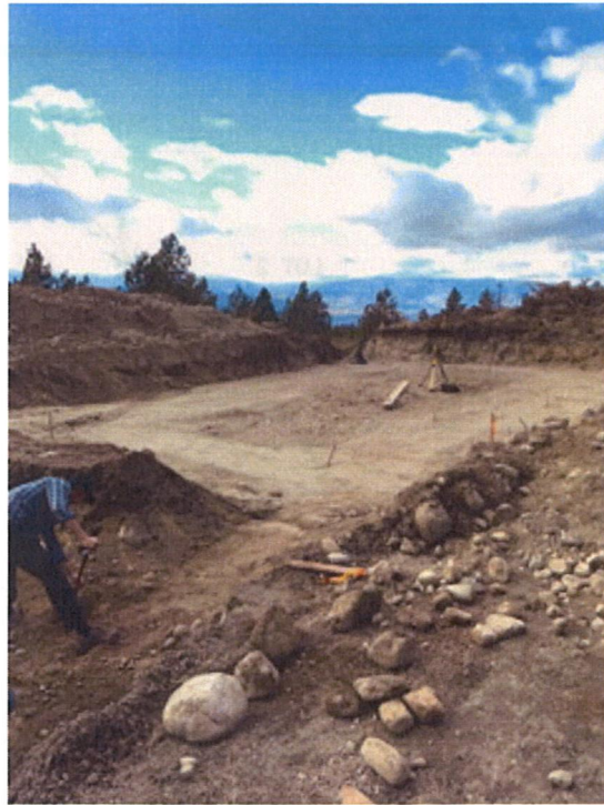
Excavation for building foundations.
