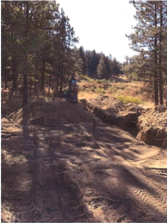
Trenching for power & well connection.
