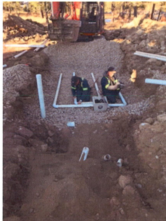
Installation of septic field
