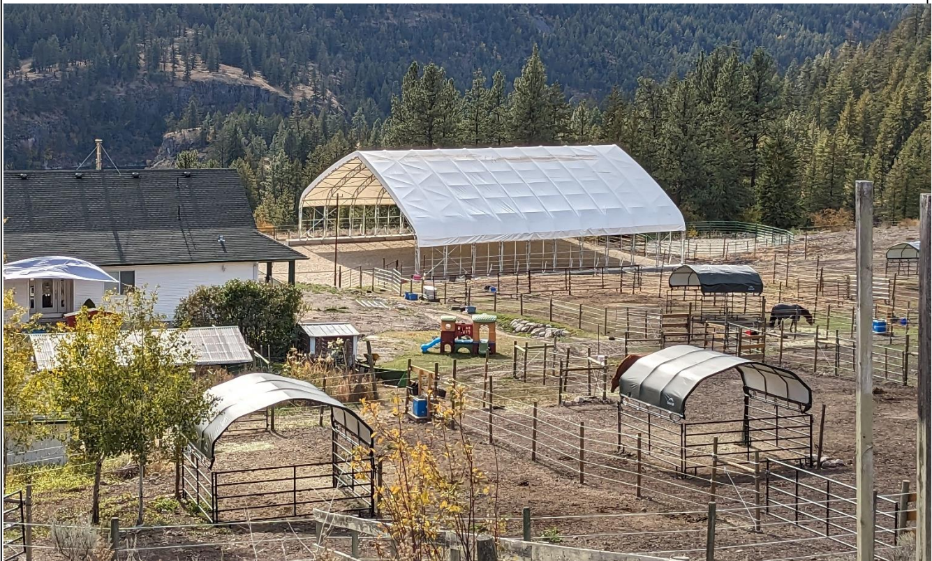
Subject Accessory Building, looking South (Photo taken October 16, 2023)
