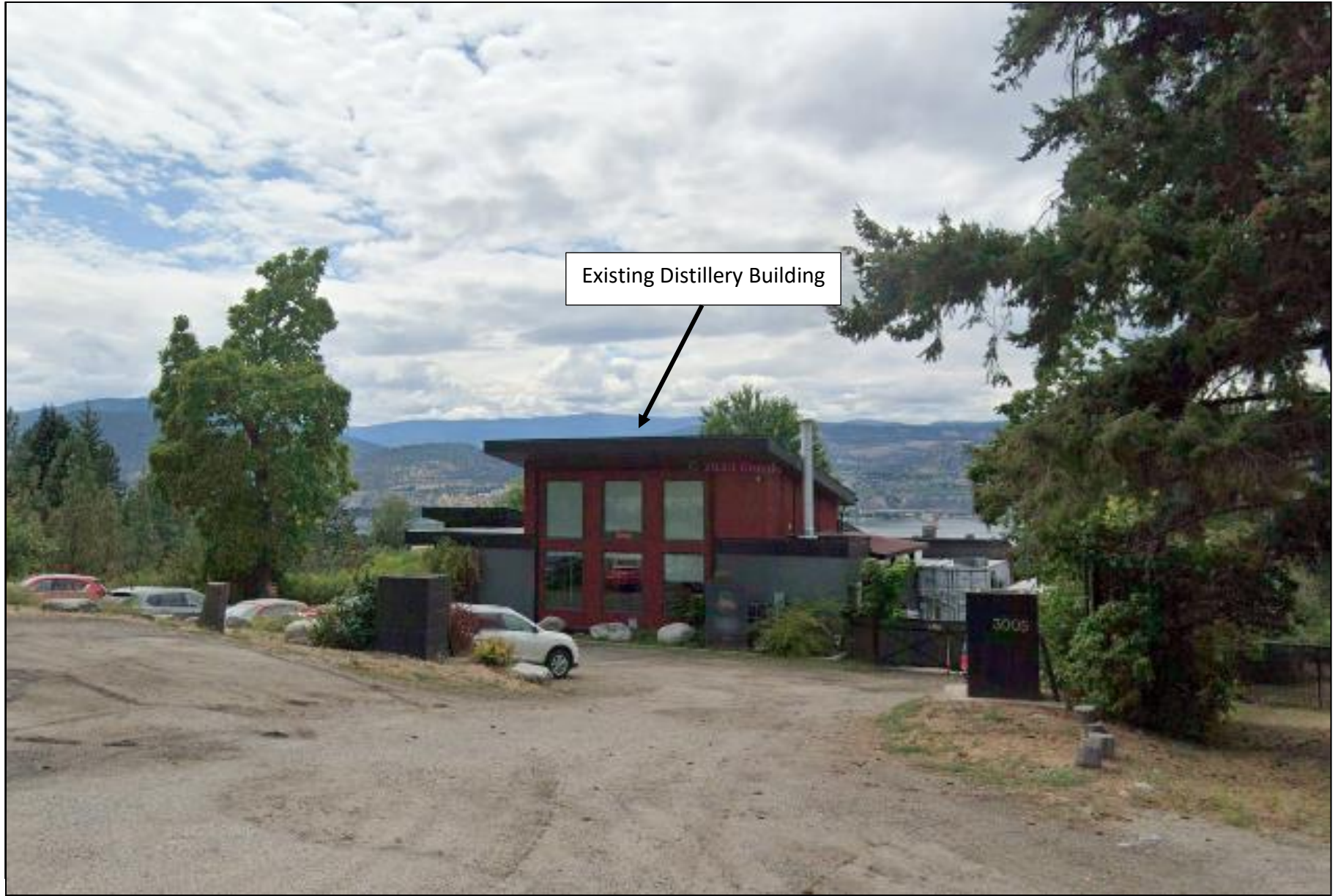
Attachment No. 3 – Site Photo (Looking West from Naramata Road)
