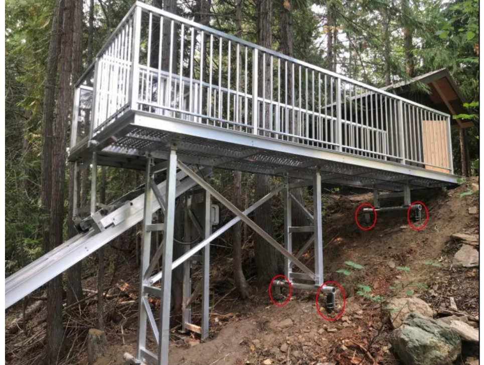
Photo 11. View of a tower bracket on two piles and their minimal permanent footprint.
