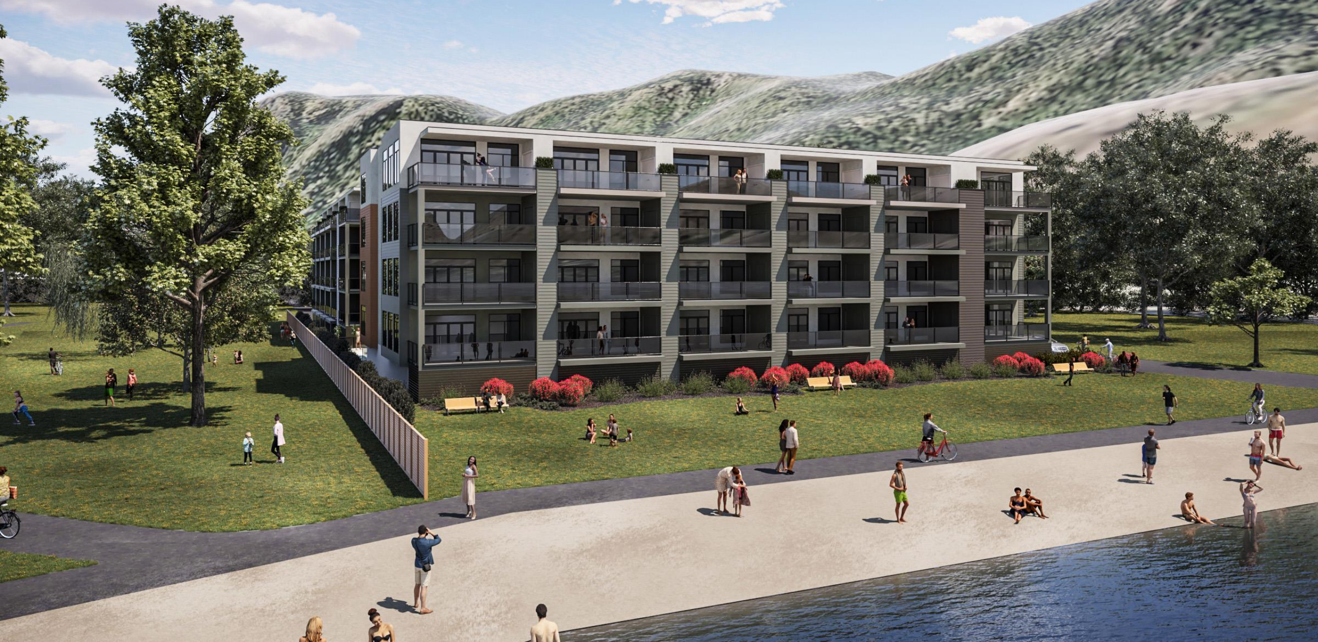
Looking south and west above Skaha Lake showing a public access lakefront pathway
