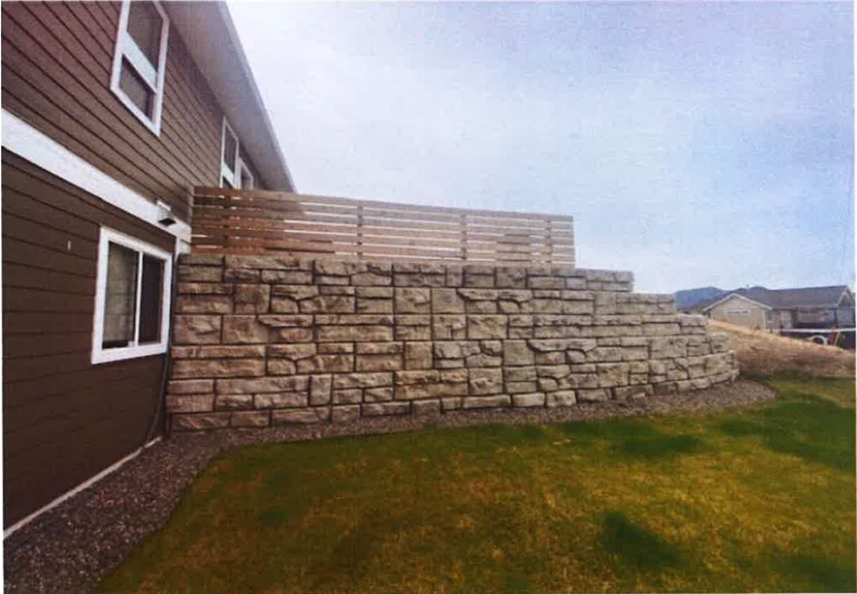
Attachment No. 2 – Site Photo (retaining wall looking south)
