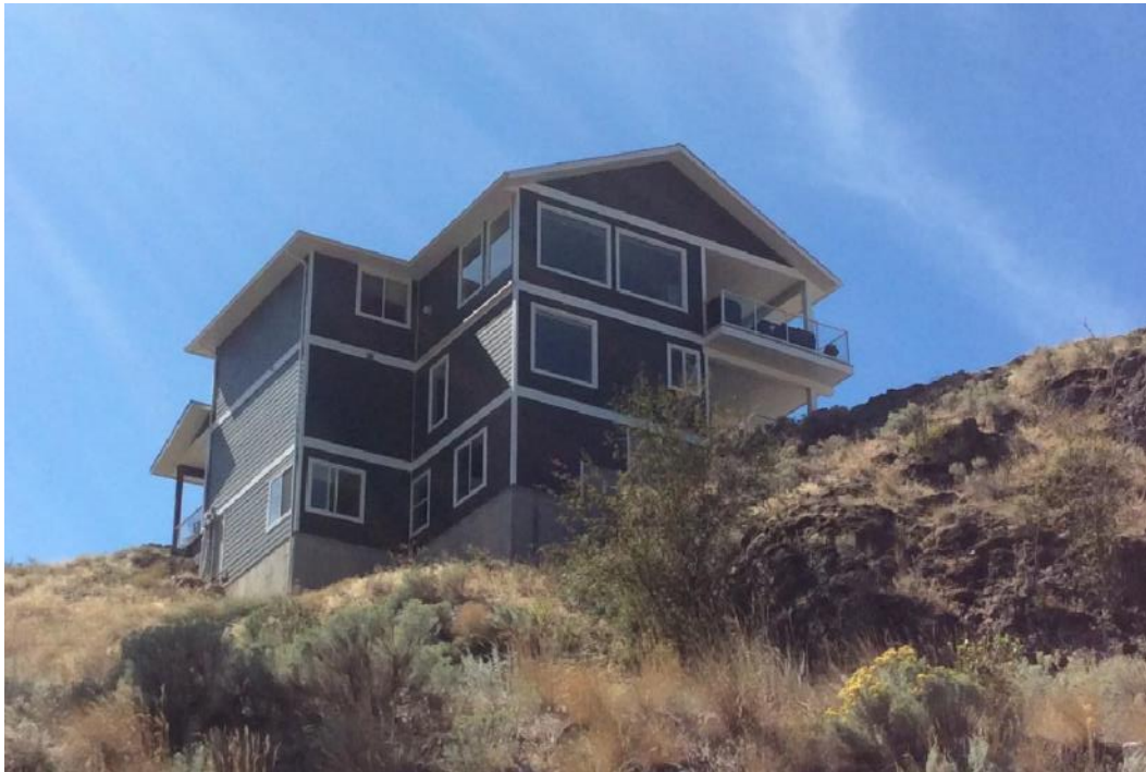
Figure 11: New homes are generally built to FireSmart building construction standards.
