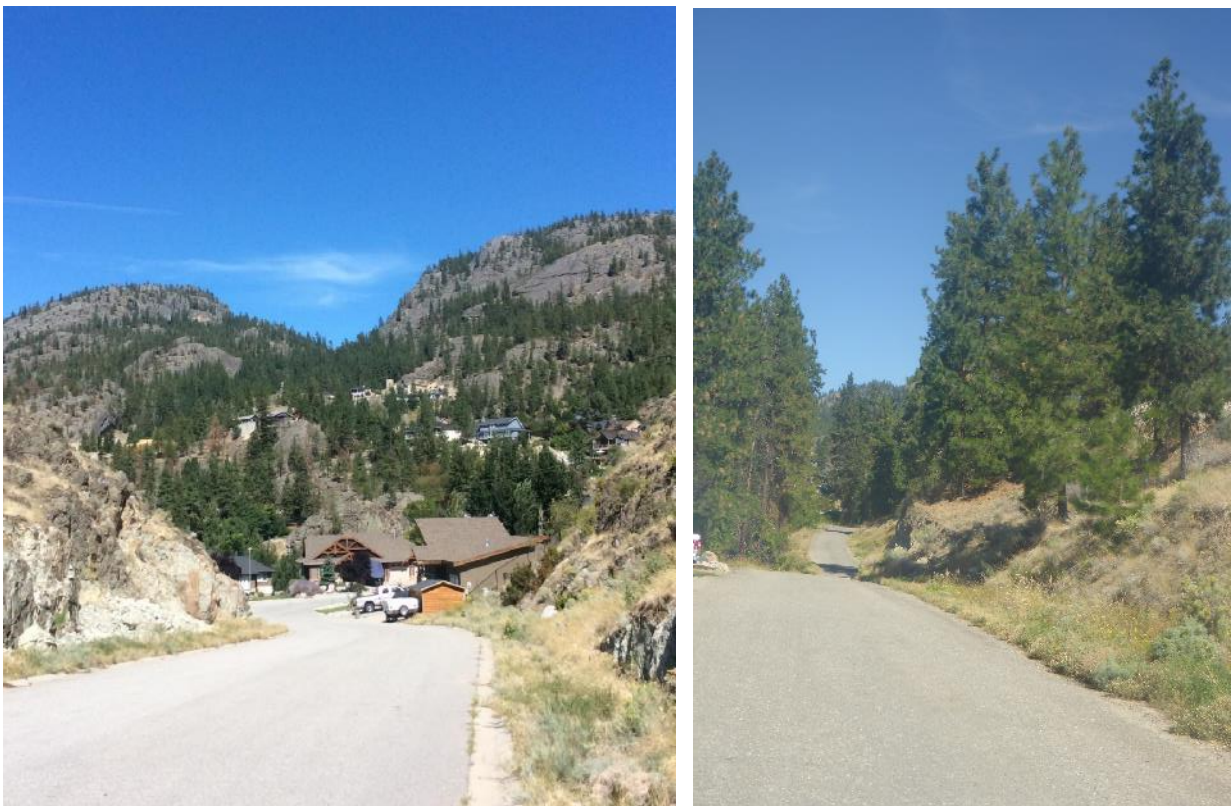
Figure 14: Dead end road at Christie Mountain Ln (L); and narrow evacuation route flanked by flammable vegetation.
