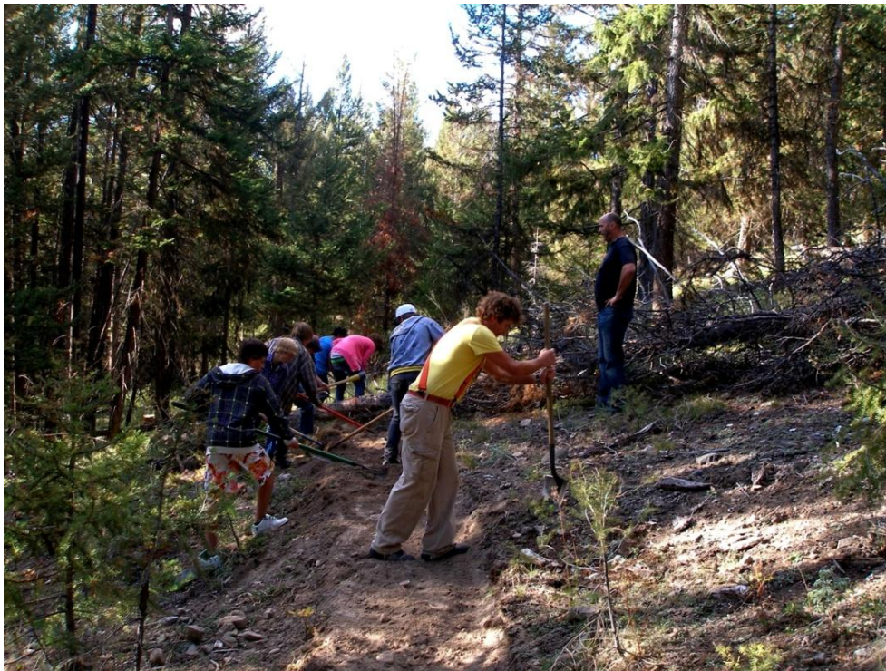
Photo 9: Trail construction in China Ridge, Princeton. Photo: DMac Trails
