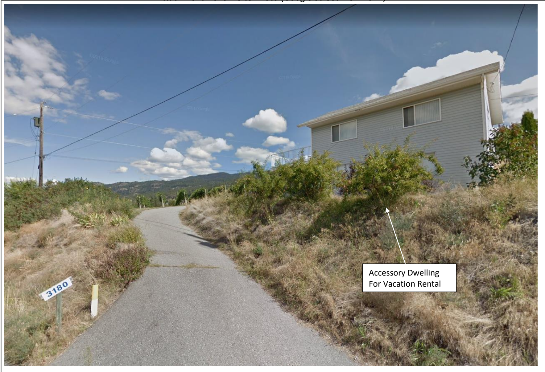
Attachment No. 3 – Site Photo (Google Street View 2012)
