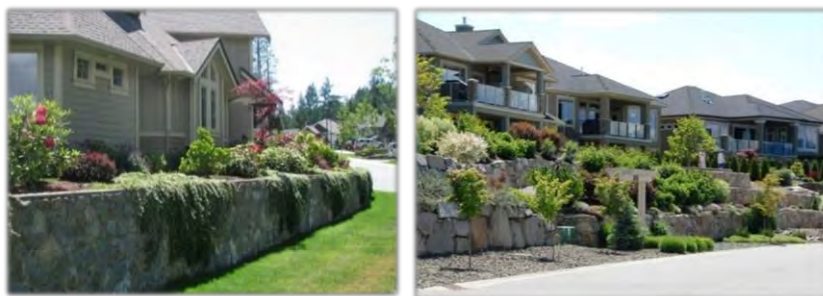
Examples of visual impact of retaining walls subdued by using context-sensitive natural materials in combination with landscaping
