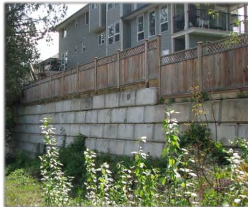
Example of Large concrete lock block that is not considered to be a context-sensitive retaining material, and if used, it should be masked or screened
