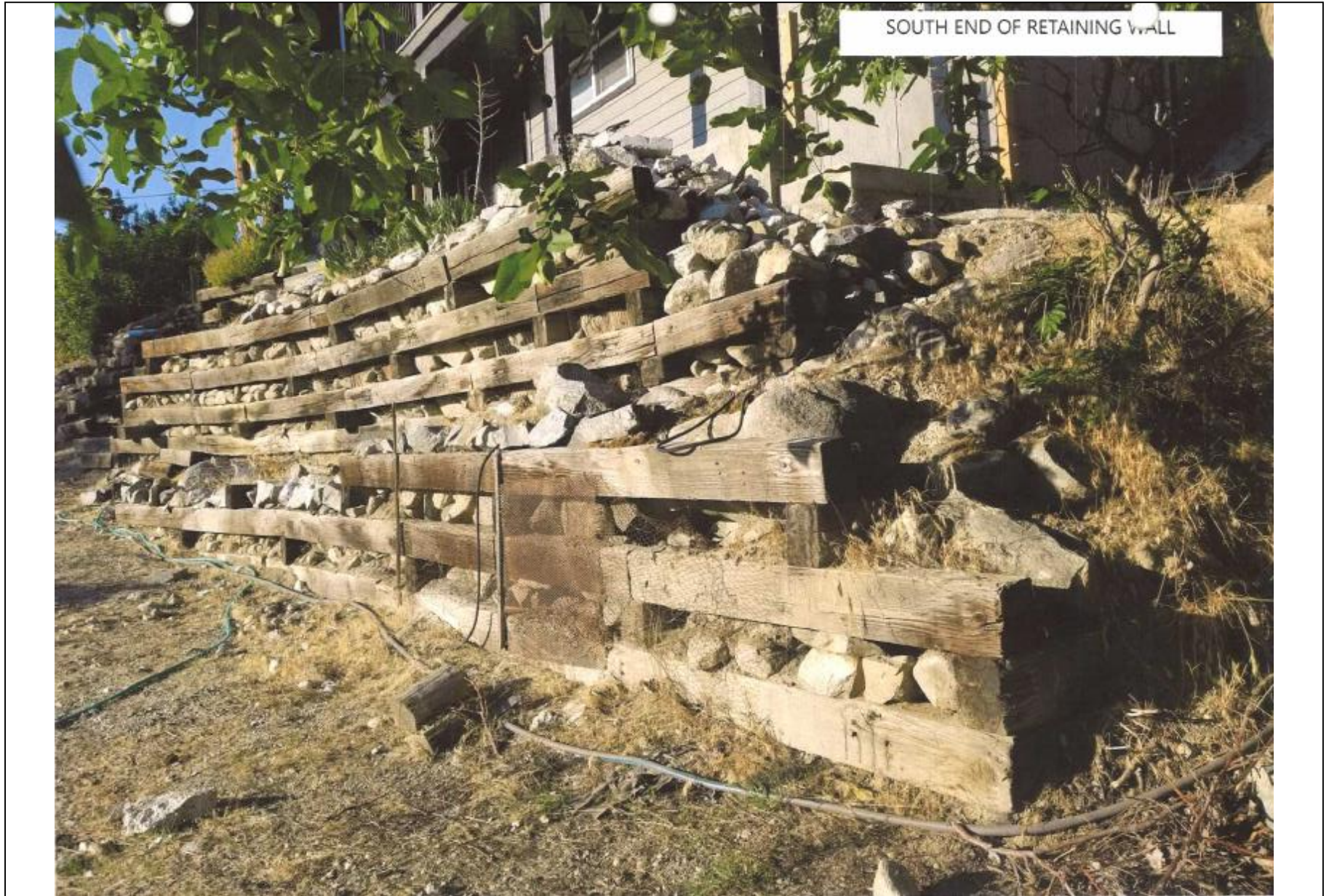
Attachment No. 3 – Site Photo (Existing Retaining Wall from South)
