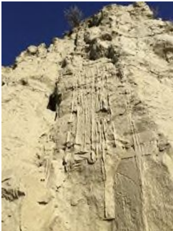
Photo 11 Silt Bluff at north end of study area – showing “wax like” flow of saturated silt
