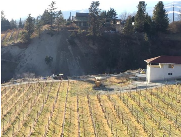
Photo 23 Fill dumping and shallow instability along gully slope (end of Moorpark Dr.)
