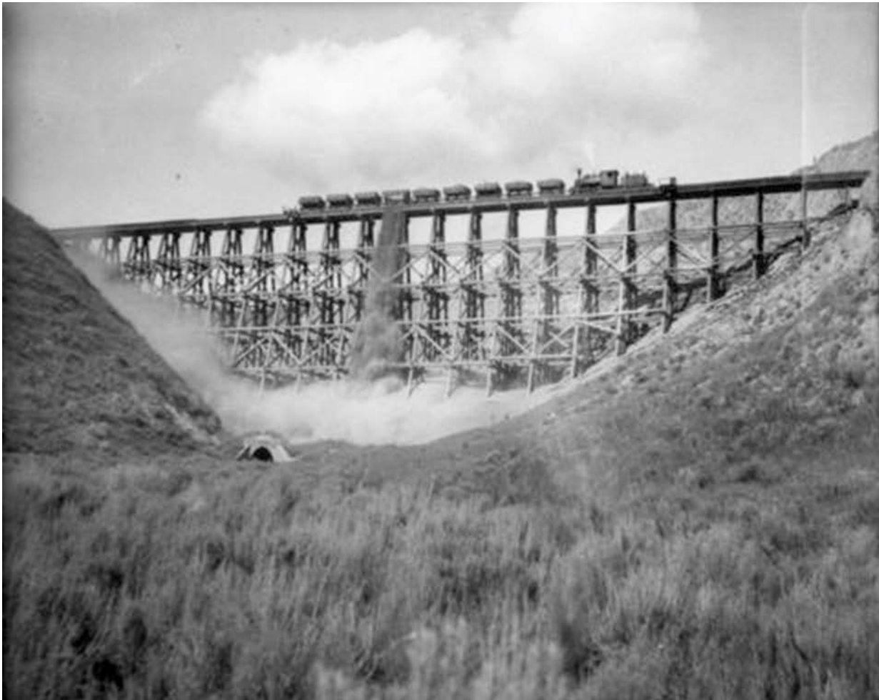
Figure 5.4.a Side dumping on KVR Trestle, at Mile 2.2 (Vancouver Archives: Item CVA 289-002.426, circa 1923) (likely located at the big gully north of Newton Drive)
