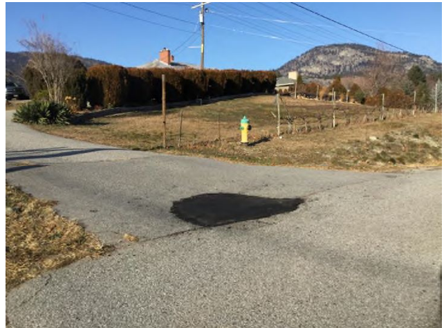
Photo 24 Recent (2019) sinkhole repair due to leaking water valve (Sparton Road)
