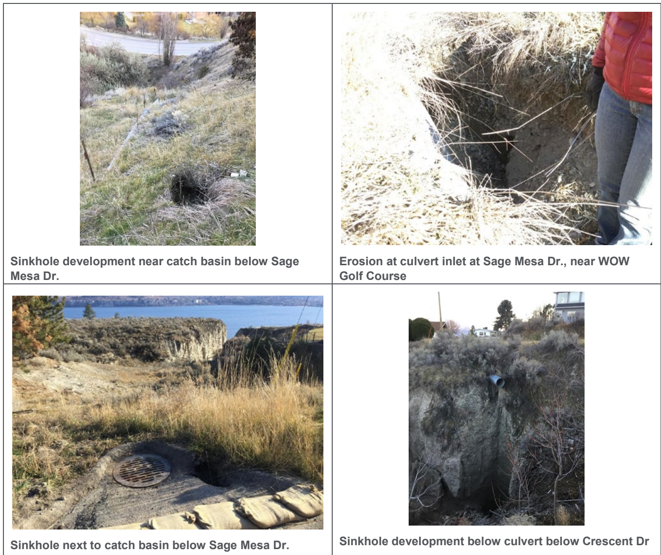
Figure 4.3.a Photographs of Example Sinkholes and Erosion Features Associated with Stormwater Management in the GWB Study Area
