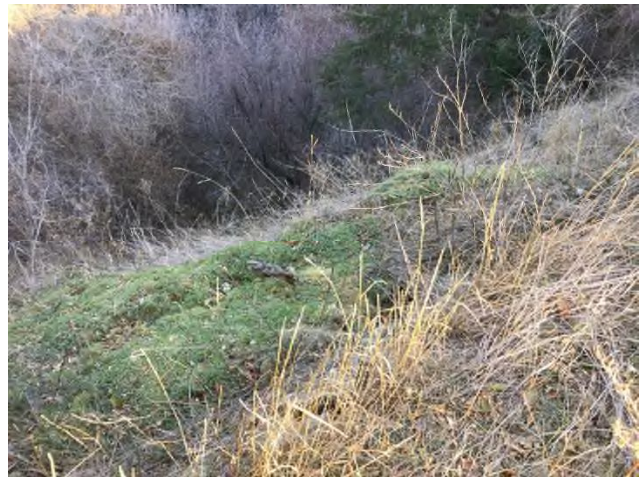
Photo 20 Tension cracks and landslide activity along crest of gully (Newton Dr and Duchess Dr.)
