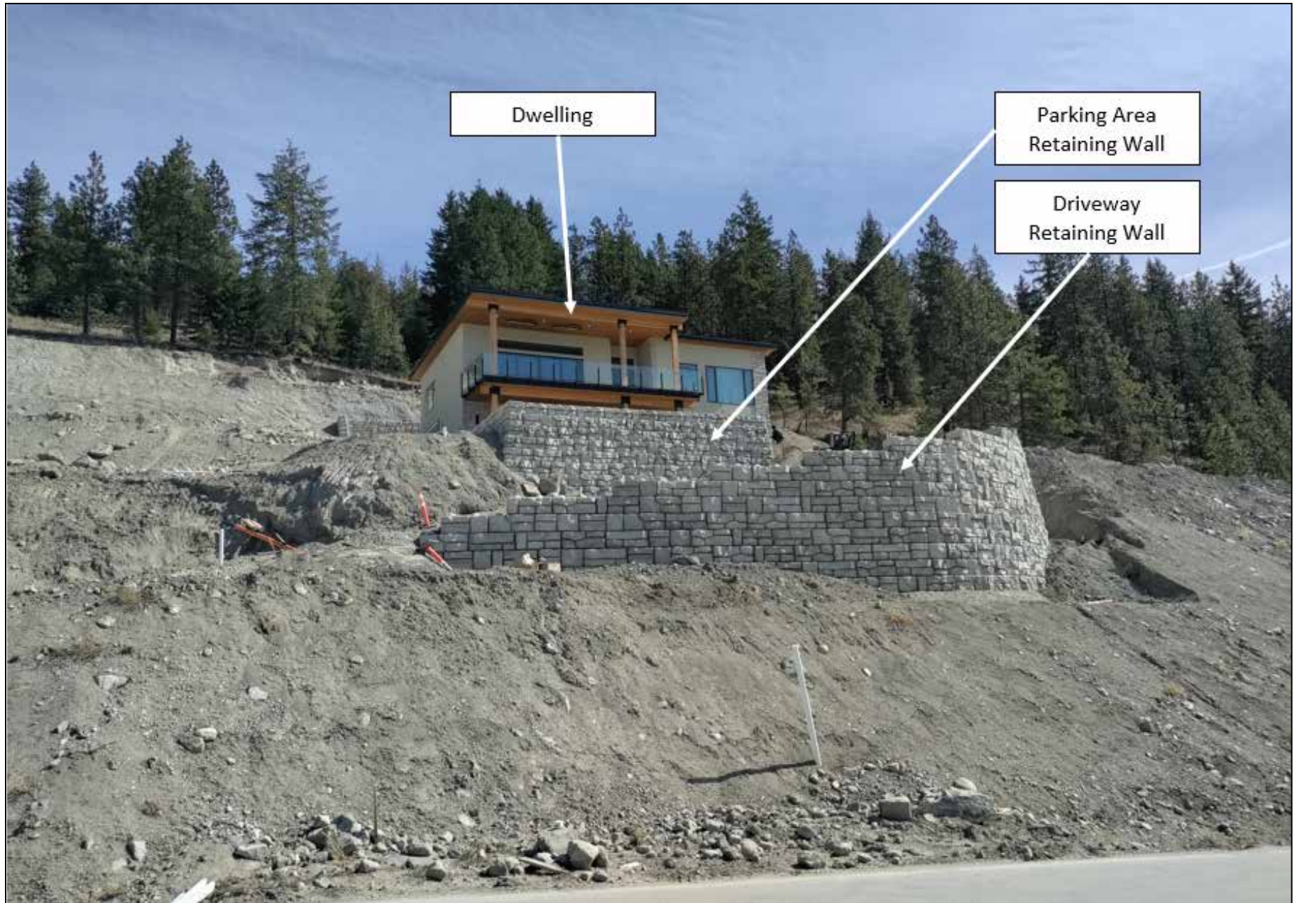
Attachment No. 1 – Site Photo (April 2021)
