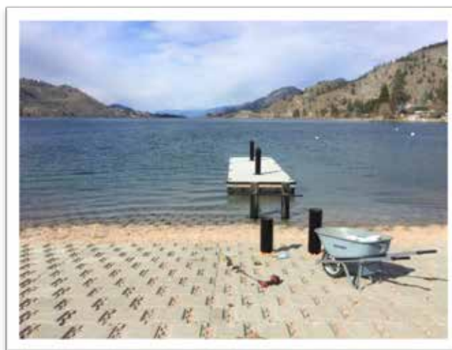
Okanagan Falls Boat Launch and Dock Project
