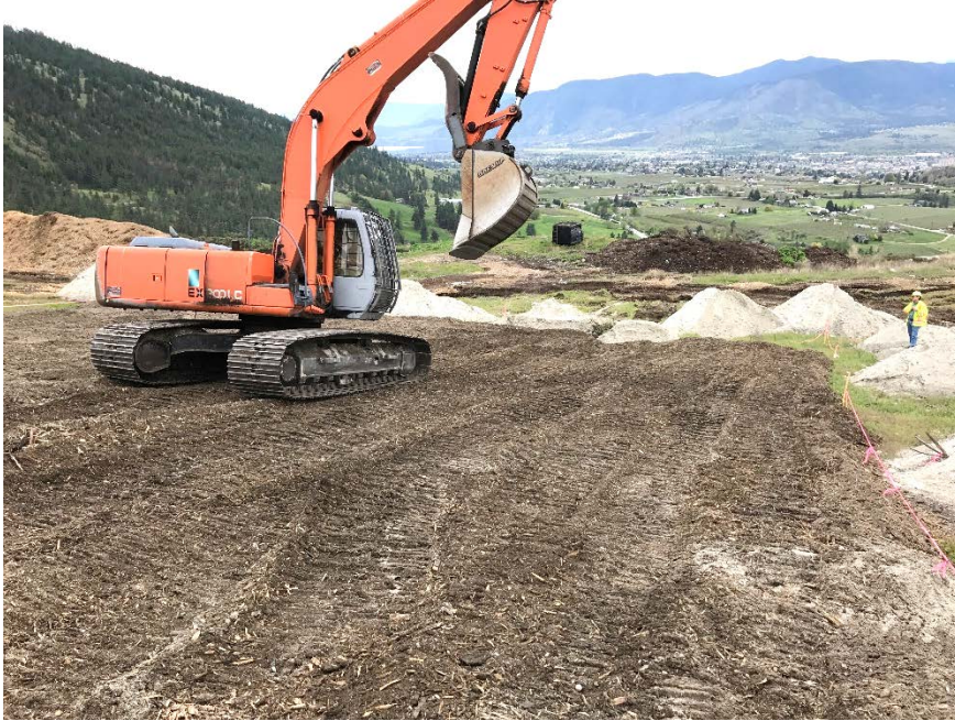
Photo 14 - Light compaction being completed on one of the three (3) test pads.
