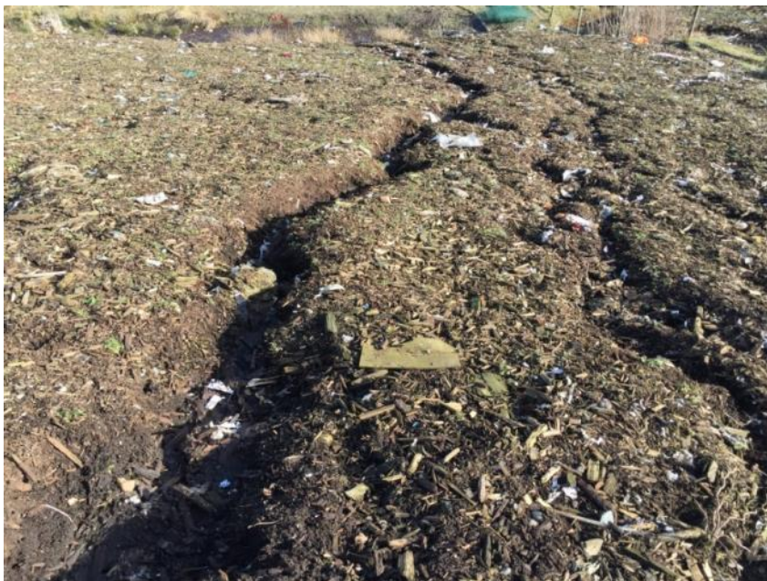
Photo 20 - Erosion channel on a biocover surface in a landfill in BC
