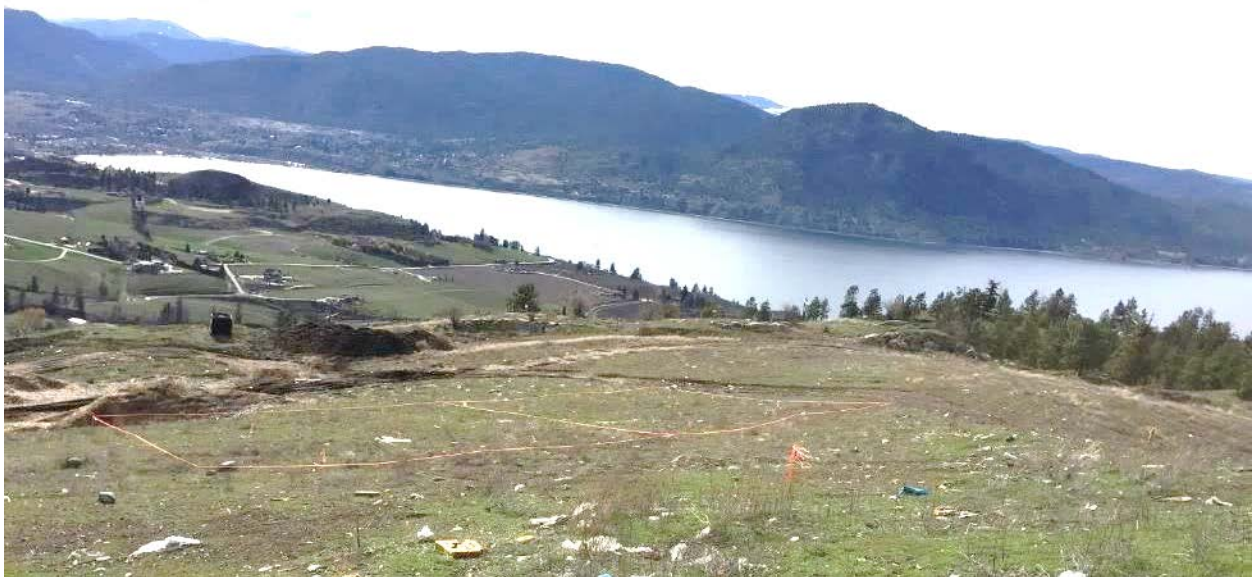
Photo 4 - TP1, TP2 , and TP3 surveyed and marked ready for Biocover construction
