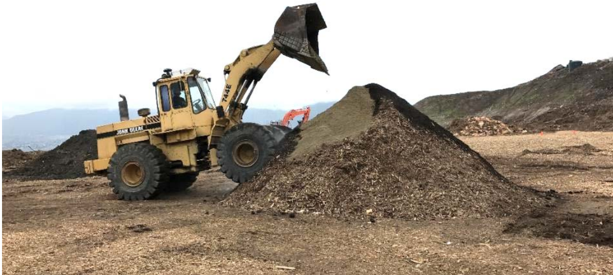
Photo 7 - ‘Pre-mix’ for each design mix. Correct quantities of each feedstock (by volume) were stockpiled by loading and high-stacking alternating materials to provide an initial rough mix.
