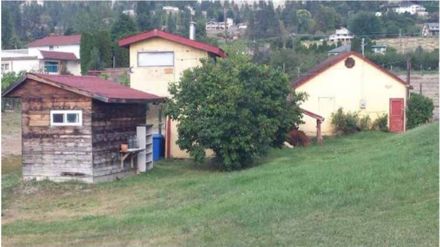
Back of Garage and Service Buildings with Apartment Above - Looking East
