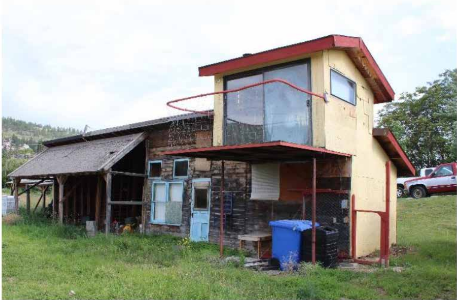
Front of Service Buildings with Apartment Above – Looking South
