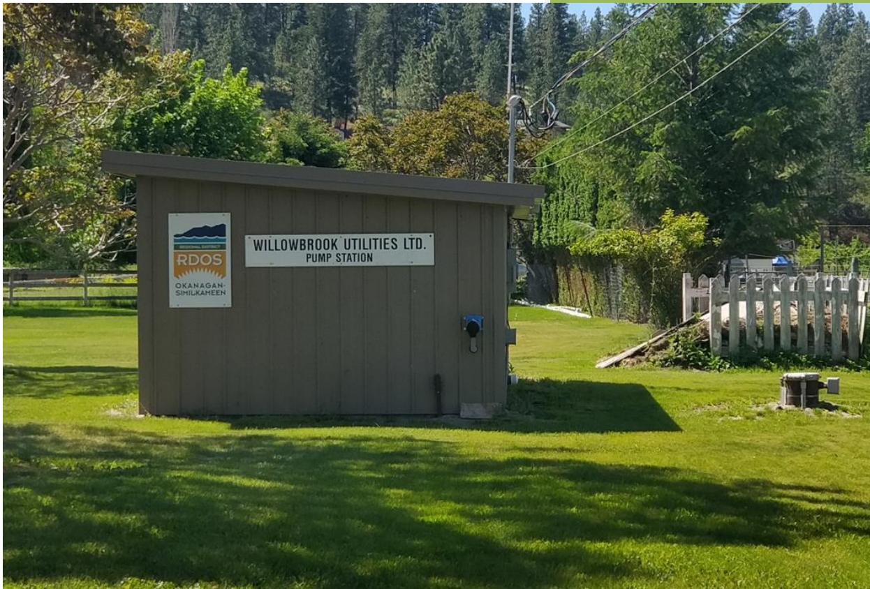
Willowbrook Well Pump Station
