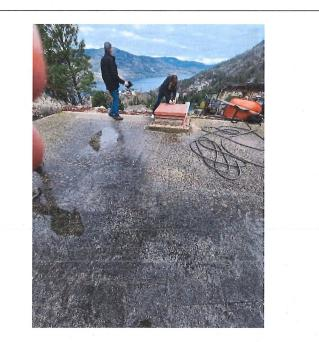
Figure 33: The roof slab of the Apple Court Reservoir is covered with lichen and moss, but generally in good condition.
