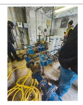
Figure 15: Sunnybrook Pumphouse: Corroded pipework and valves, untidy tubes, dirty ceiling
