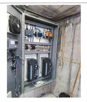
Figure 17: Sunnybrook Pumphouse: 600 Volt Variable frequency drives (VFDs) and programmable logic controller (PLC) in the same box
