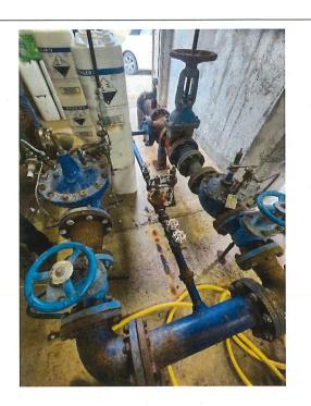
Figure 16: Sunnybrook Pumphouse: Corroded steel pipework and corroded valves
