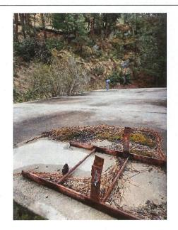
Figure 31: Sunnybrook Reservoir: Corroded steel ladder
