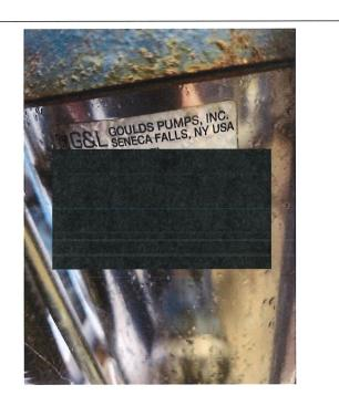
Figure 24: Christie Mountain Pumphouse: Corrosion visible on pump electrical motor frame
