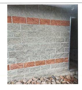
Figure 25: Apple Court Pumphouse: Cinder block walls are generally in a good condition.
