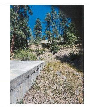
Figure 29: Sunnybrook Reservoir: Top of the concrete walls and roof slab on the left; stormwater channel on the right
