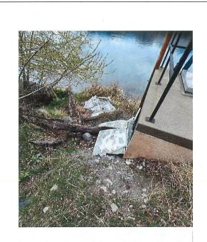
Figure 9: Lakeshore Pumphouse: Disintegrating outer walls.
