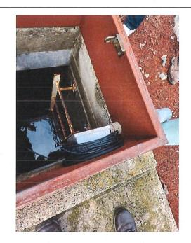
Figure 32: Apple Court Reservoir: Internal ladder shows signs of corrosion.
