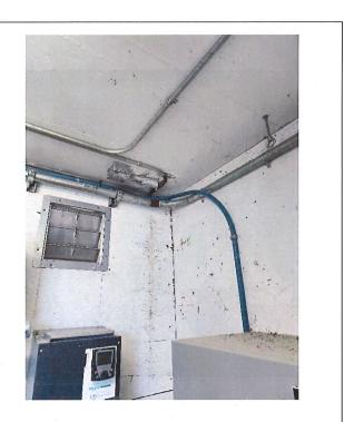
Figure 14: Lakeshore Pumphouse: Bottom Level: Leak through roof
