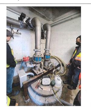
Figure 8: Lakeshore Pumphouse: Wet well and pump headers
