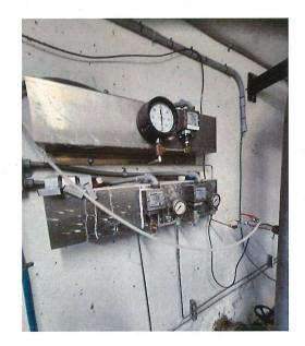
Figure 11: Lakeshore Pumphouse: Bottom Level: Mechanical pressure gauges and tubes
