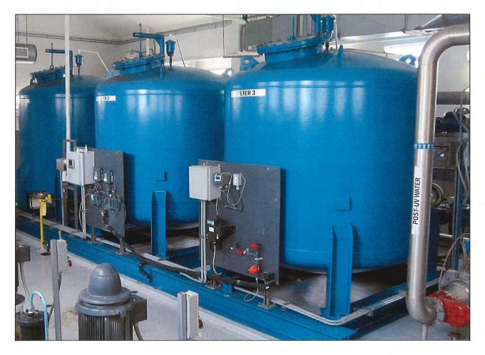
Figure 34: A typical pressure filter installation
