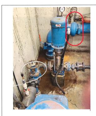
Figure 23: Christie Mountain Pumphouse: Pressure Reducing Valve requiring testing and refurbishment.
