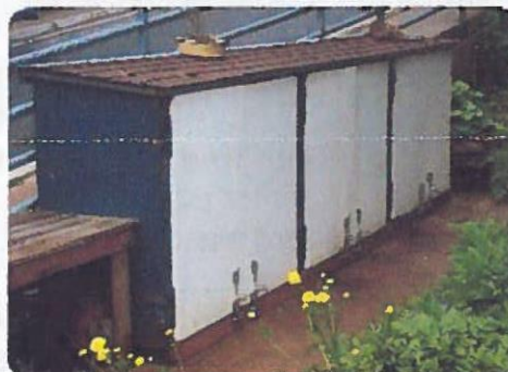
Home constructed Garbage Enclosure with metal seams and heavy duty handles
