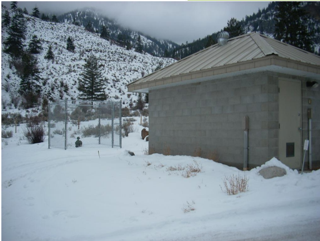
Olalla Well Pump Station
