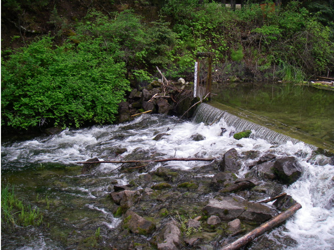
All debris below the weir was removed
