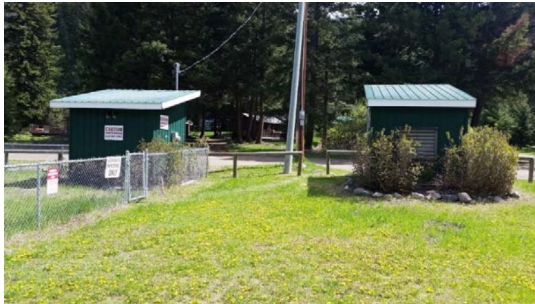
Pumping building (left) and generator building (right) – built in 2002
