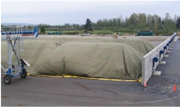
Photo 3.2: Membrane Covered Aerated Static Pile
