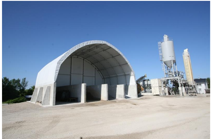
Figure 3.1: Example of clear span structure
