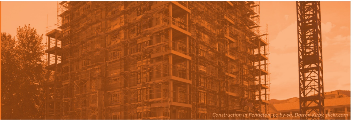
Construction in Penticton, cc-by-sa, Darren Kirby, flickr.com
