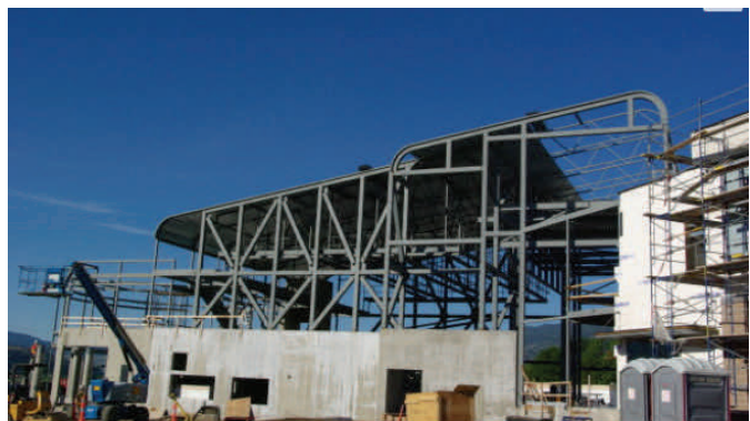
Construction began on the new Frank Venables Theatre in Oliver
