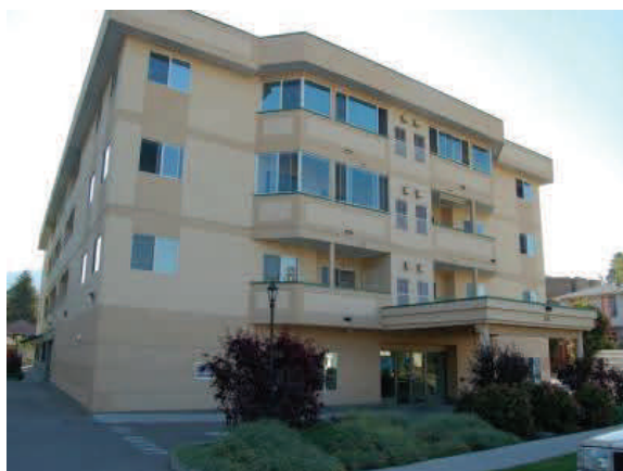
Multi-family units may serve to increase housing affordability and variety. This is a Kiwanis housing project in Penticton.
