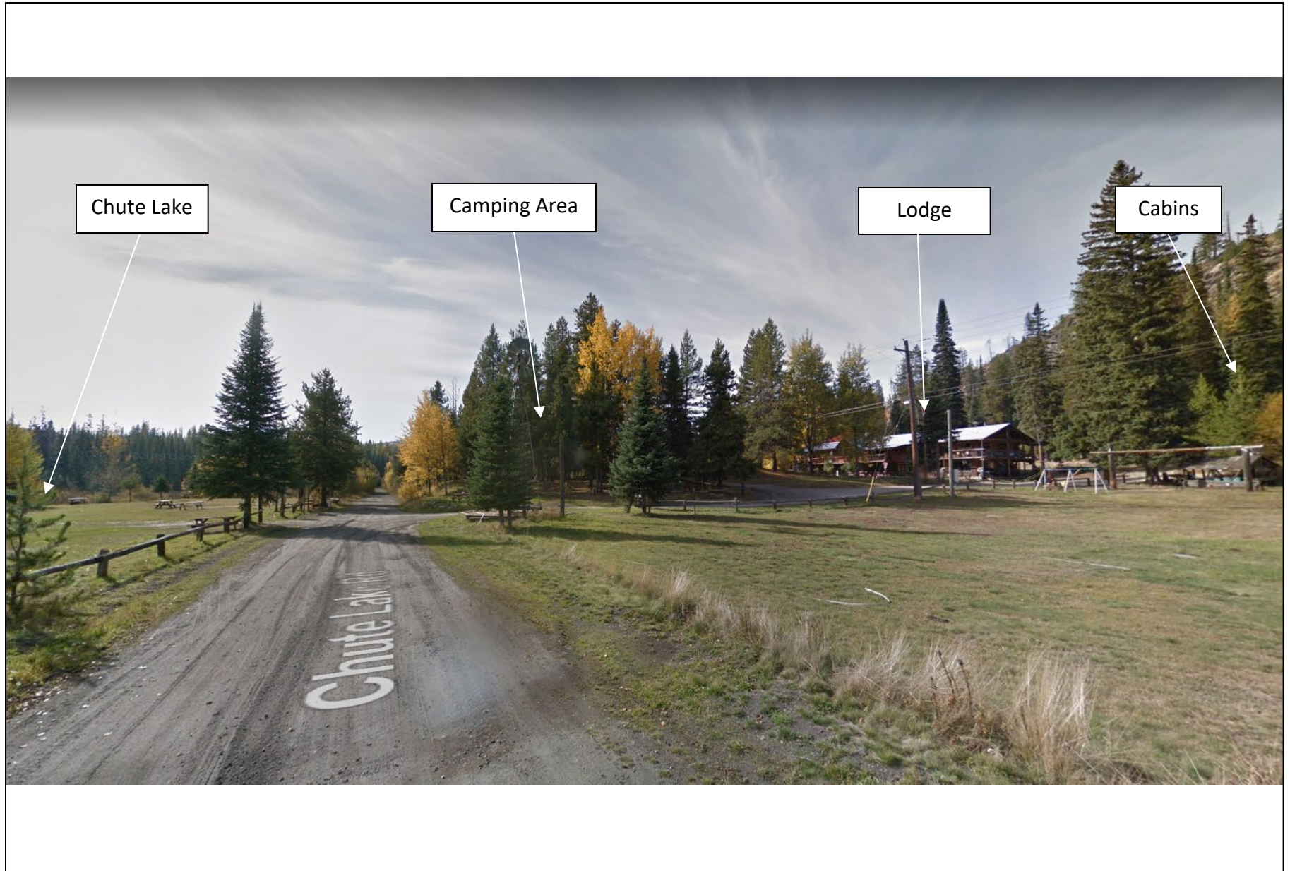
Attachment No. 3 – Site Photo (Google Street View 2014 looking south)
