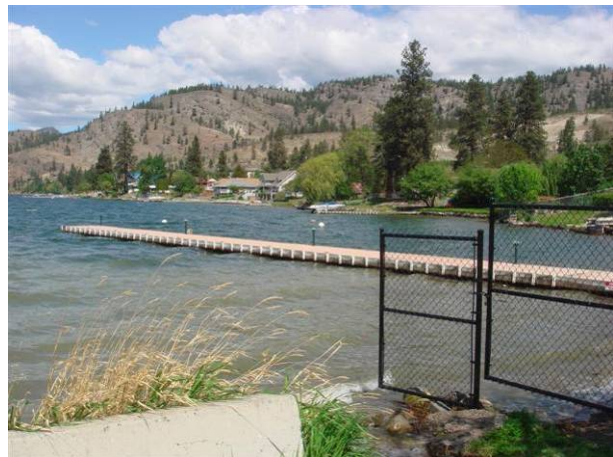
Photo 17: Private dock for condominium development on east side of the Main Street boat launch (Segment 32).
