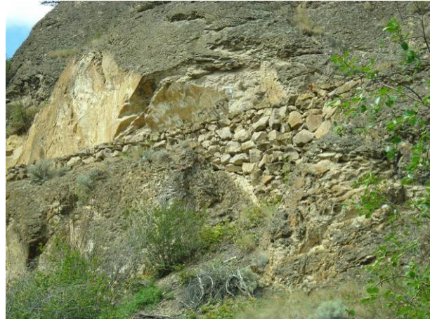
Photo 33: Rock fill along old trail visible from KVR trail (Segment 24).
