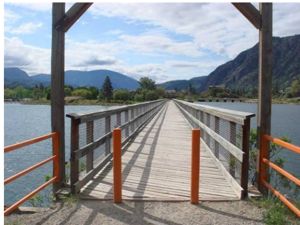
Photo 52: The KVR trestle at Okanagan Falls (Segment 29).
