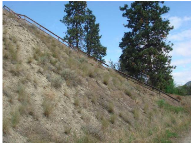
Photo 27: Stairway that provides access from a residential development to KVR Trail and Skaha Lake shoreline (Segment 22).
