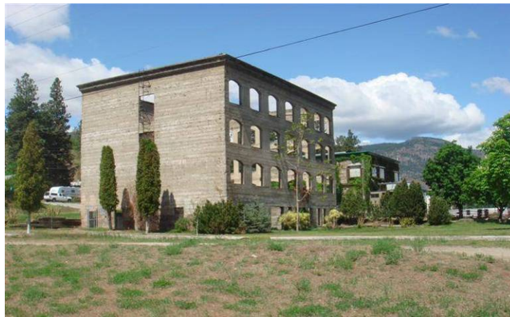
Photo 45: Kaleden Hotel Park (Segment 18).
