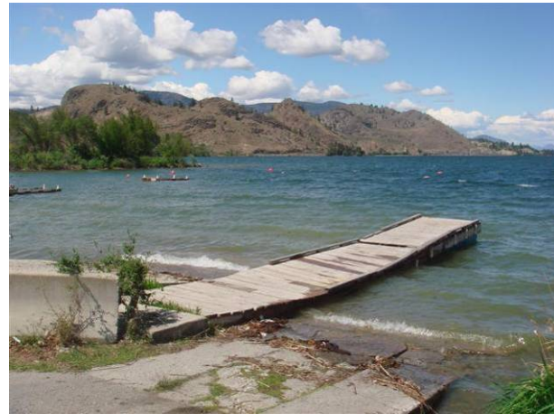
Photo 13: Public dock at the Okanagan Falls boat launch (Segment 32).
