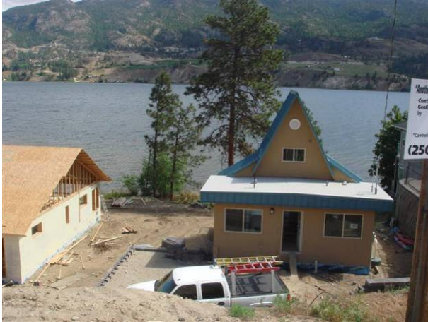
Photo 36: Example of single family land use in a Low Density Residential zone (RL1) on the shoreline in Kaleden (Segment 20).
