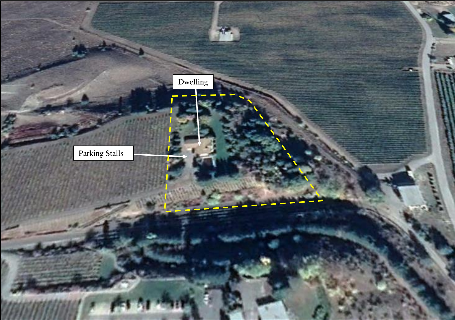
Attachment No. 5 –Photo (Google Earth)
