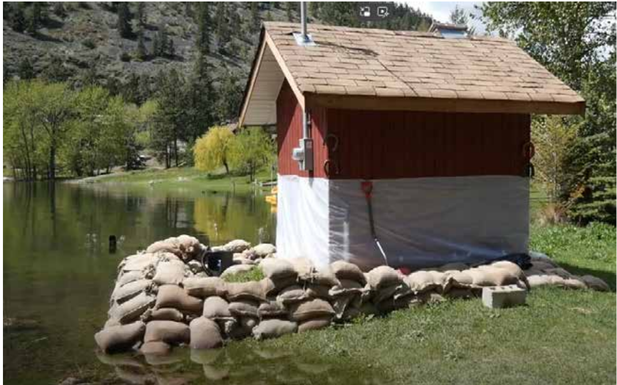
Lower Nipit well pumphouse during flood event 2021
