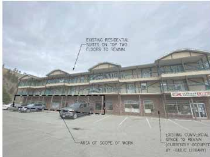
EXISTING BUILDING (NORTH ELEVATION) DATE: 10/19/20
